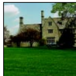
The structurally impressive Hartwood Mansion is also home to many County assets and historical treasures.
