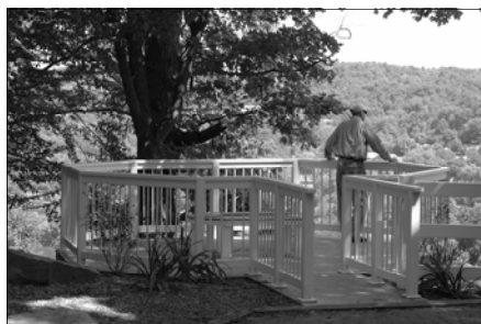
Watts Memorial Overlook Expansion
