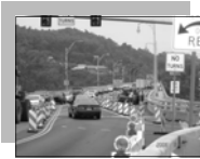
Homestead Grays Bridge Rehab Project Reaches First Milestone
