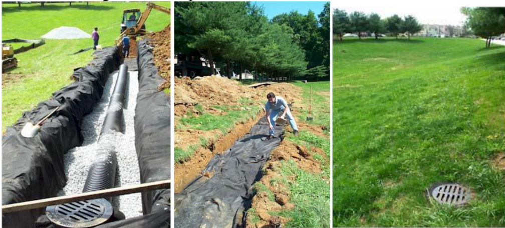
Figure 3: Example of Infiltration Trench Installation
