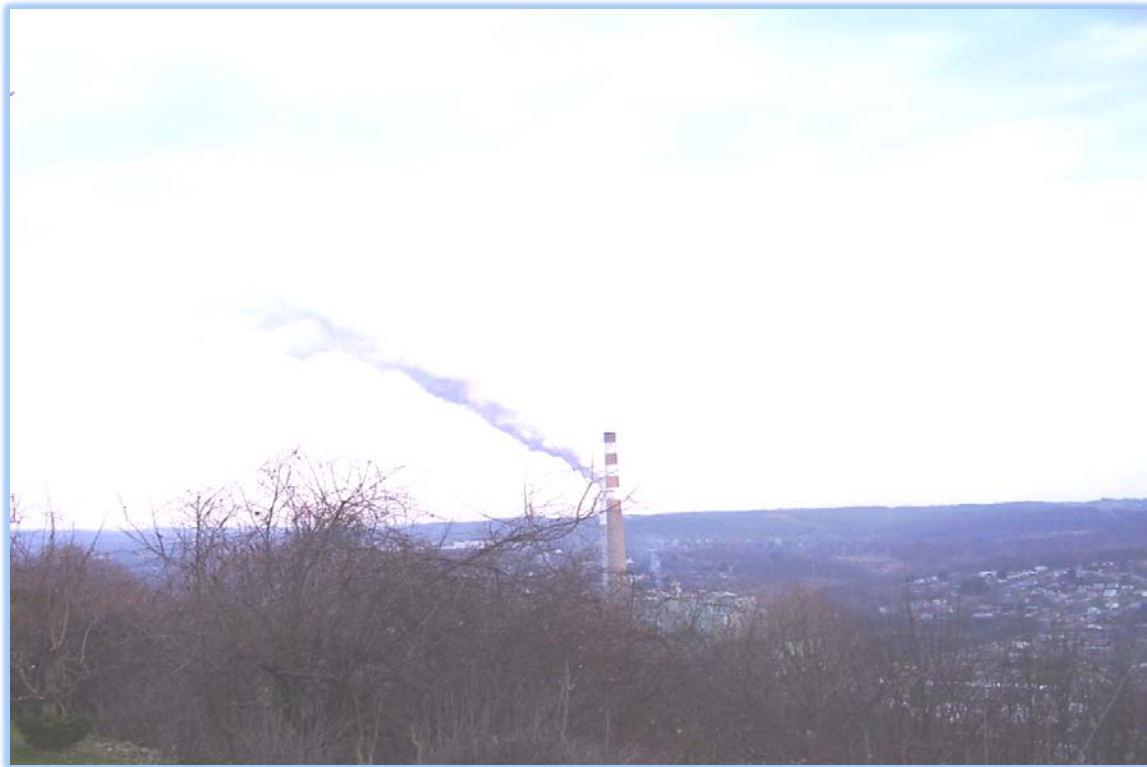
CHESWICK POWER PLANT STACK
