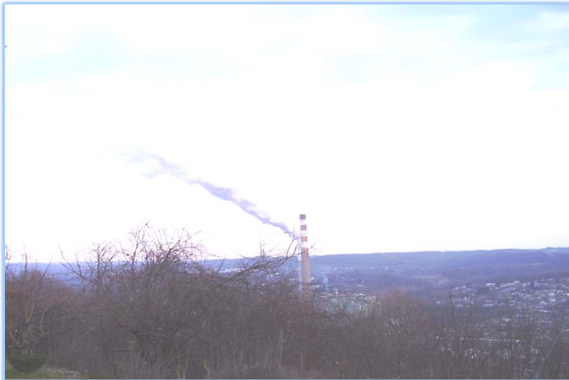
CHESWICK POWER PLANT STACK
