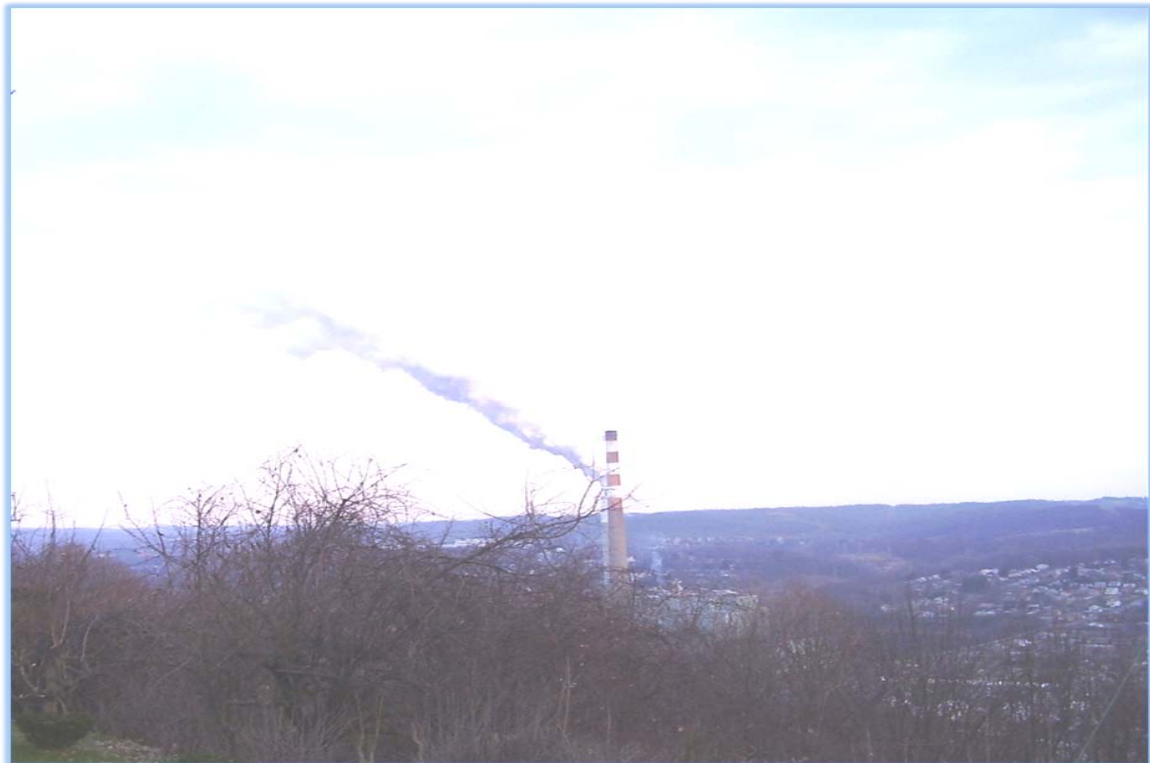
CHESWICK POWER PLANT STACK
