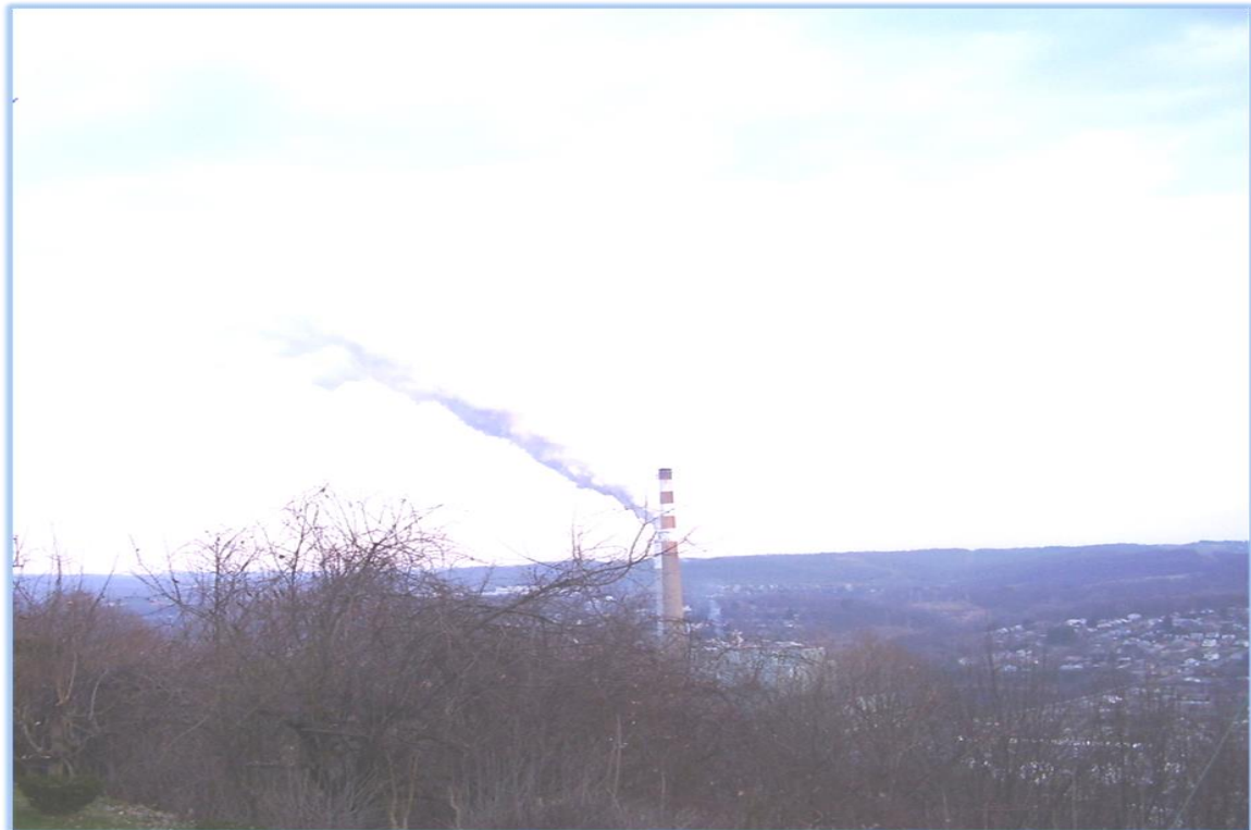
CHESWICK POWER PLANT STACK
