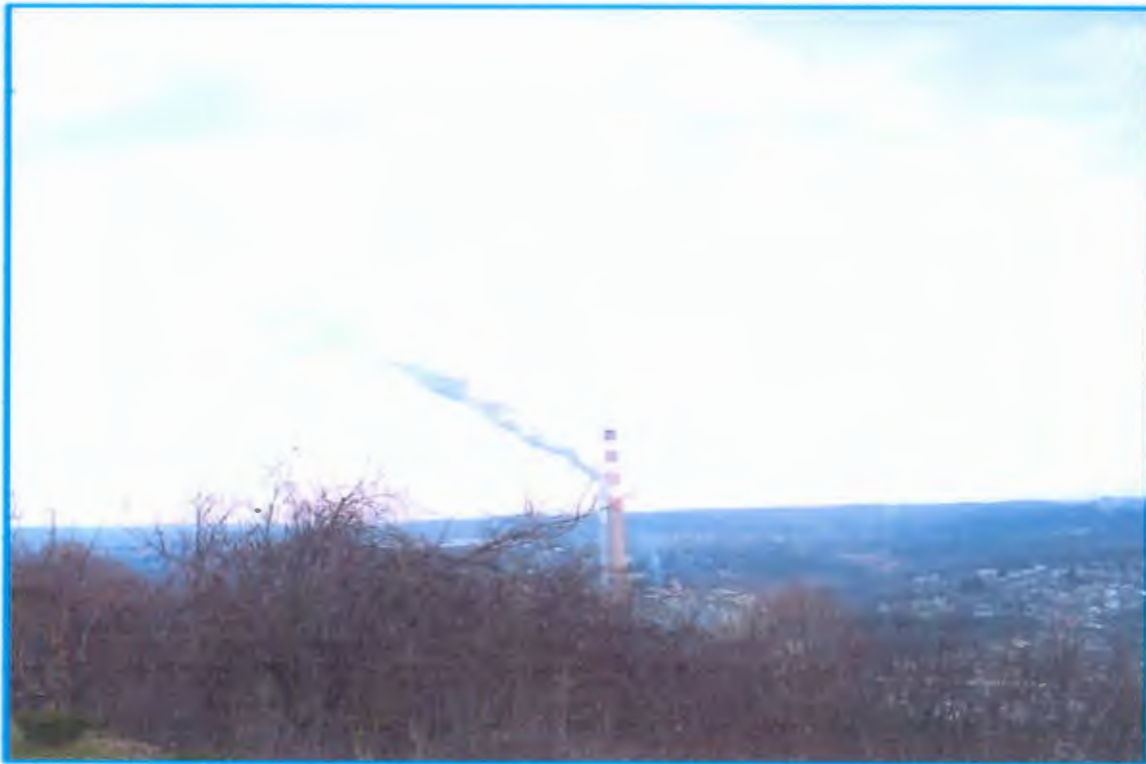
CHESWICK POWER PLANT STACK
